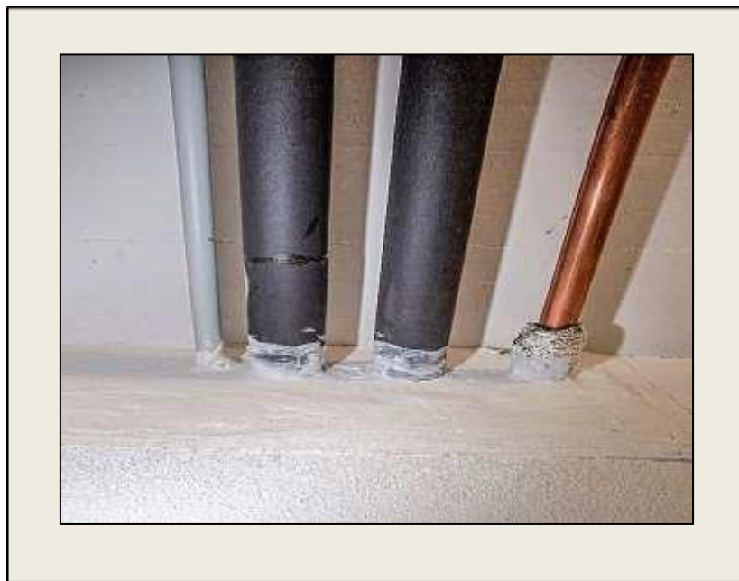
Figure 20 Fire Stopping of Pipe Penetration Wall
