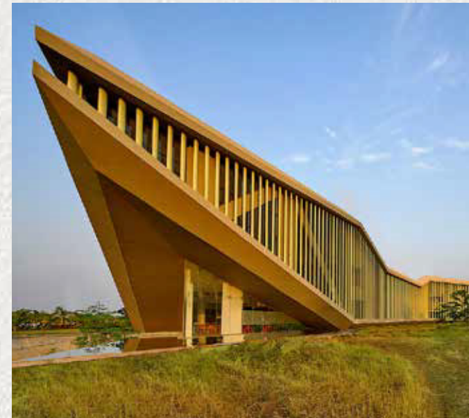
The Courtyard, Raipur
